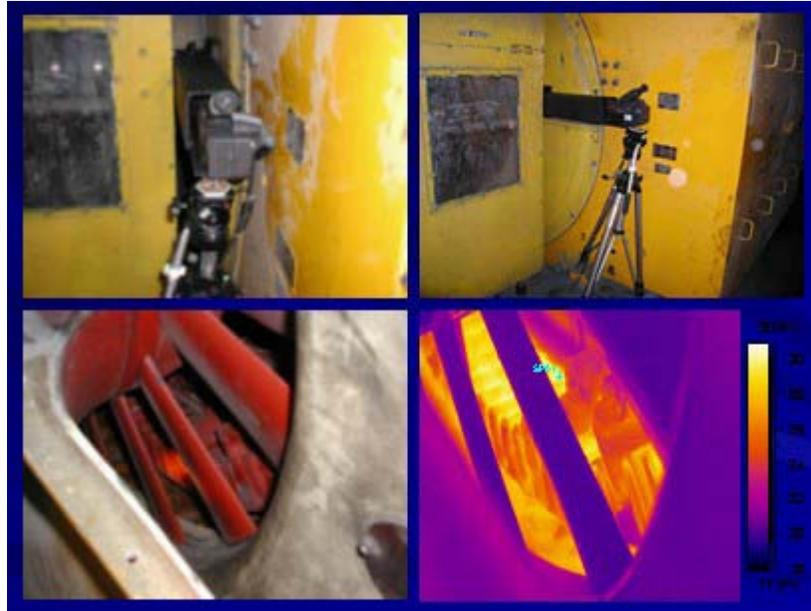
**Fig. 6 - Thermographic Condition Monitoring of SSBFP Motor**
