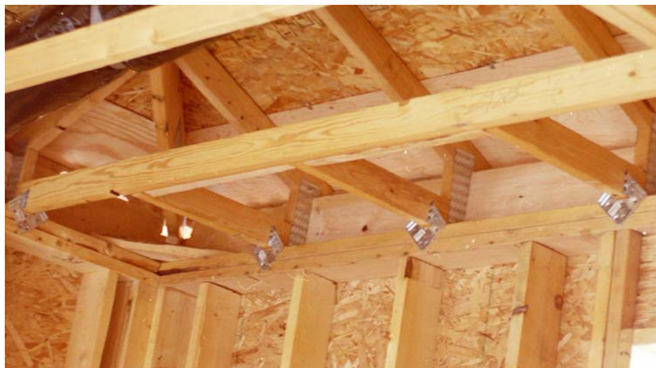
Figure 5. Metal-plate-connected wood trusses.
