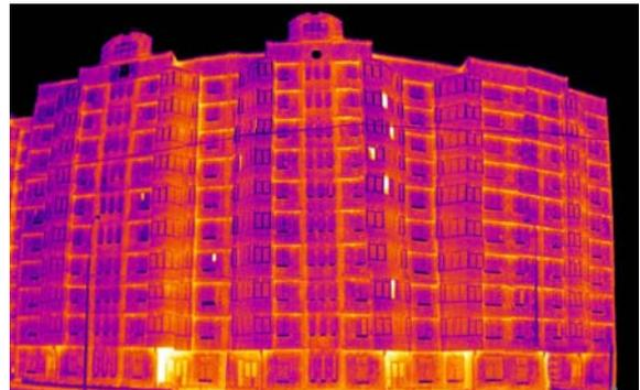
Fig.4. A typical thermogram of outdoor guarding construction of a building.
