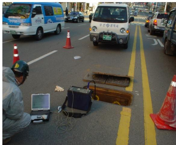
Figure 5. Guided wave inspection for buried heat exchange facilities
