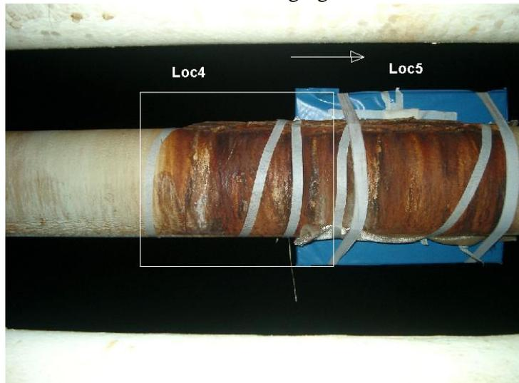
Figure 3. Pipe with scaling and wall loss
