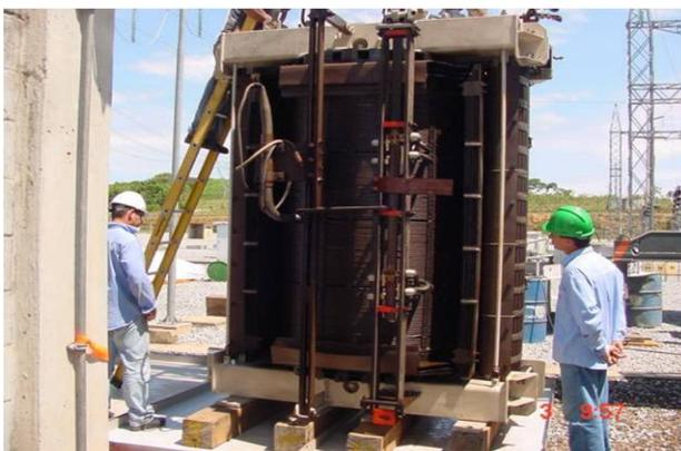
**Figure 3 – Inspection of the autotransformer after removal of the tank**
