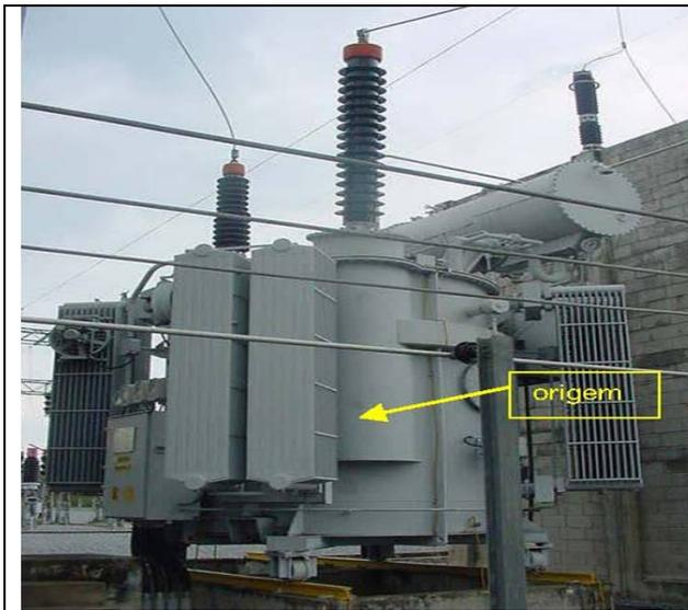
**Figure 1 – Monophase Autotransformer 230/138 kV, 50 MVA**
