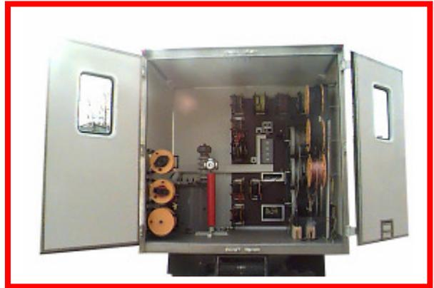
**Fig.4. High-Voltage Compartment**
