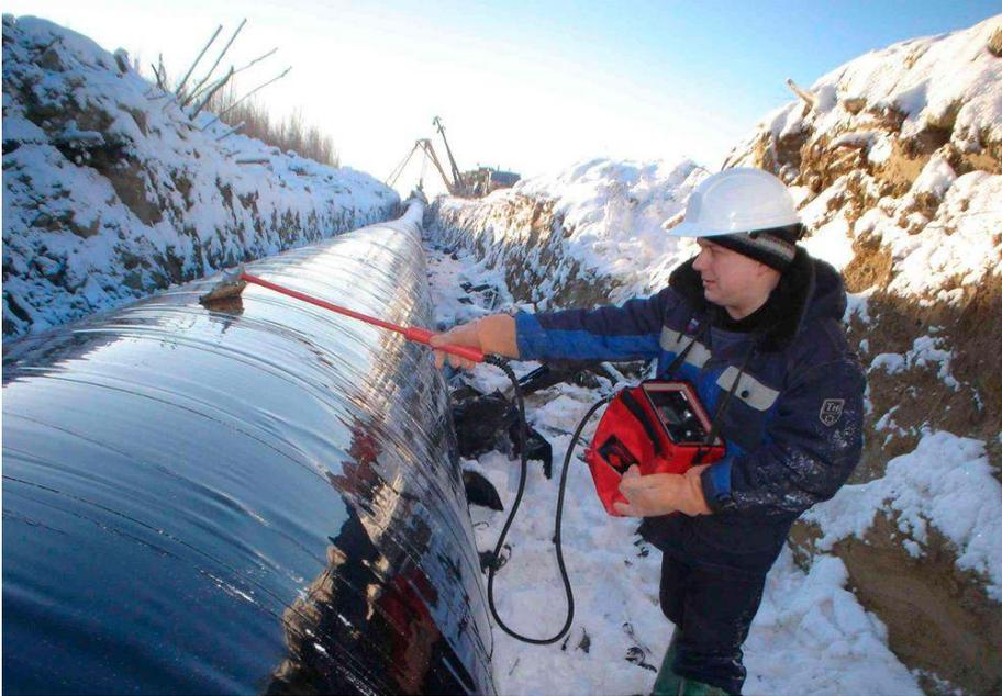
Fig.5. Electric spark defectoscope
