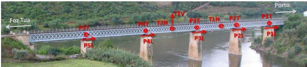
Figure 8: Degrees of freedom instrumented with accelerometers.
