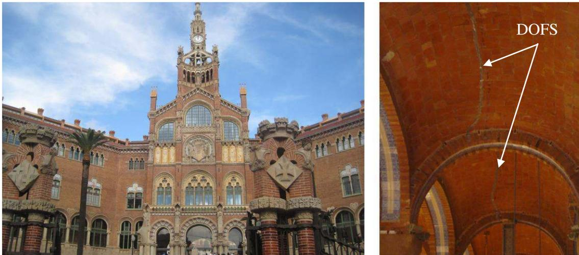
Figure 5: Sant Pau Hospital, Barcelona (left) and DOFS installed on the masonry vaults (right) [15]
