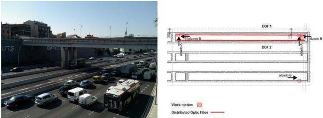
Figure 2: Sarajevo Bridge at Barcelona (left) and general scheme of DOFS monitoring scheme (right) [15]
