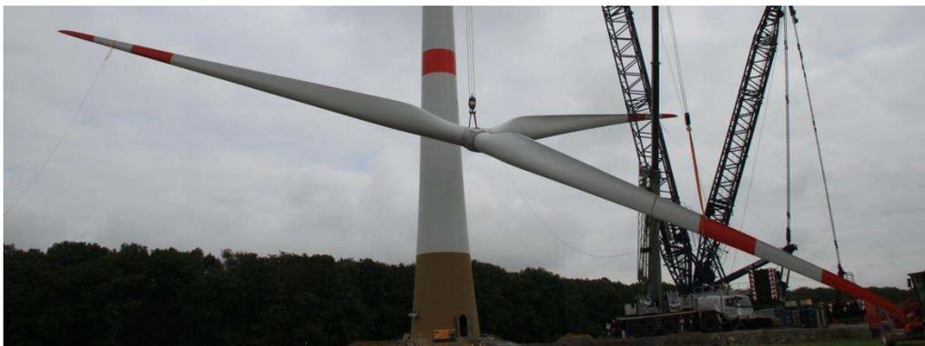
Figure 4: Rotor blade of wind turbines are typical SHM-structures. The length of the blade is about 59 m, the diameter of the rotor is 117 m
