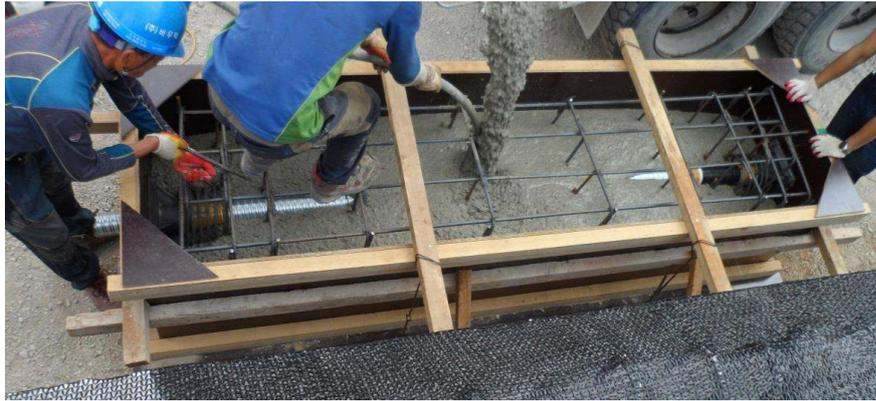
Figure 5: Concrete casting in test specimen
