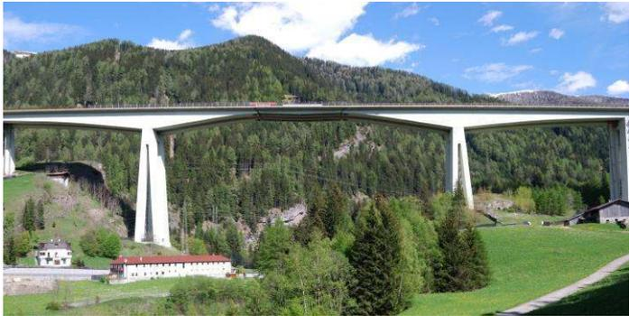
Figure 1: Main span of Colle Isarco Viaduct; left pier is #8, right is #9.
